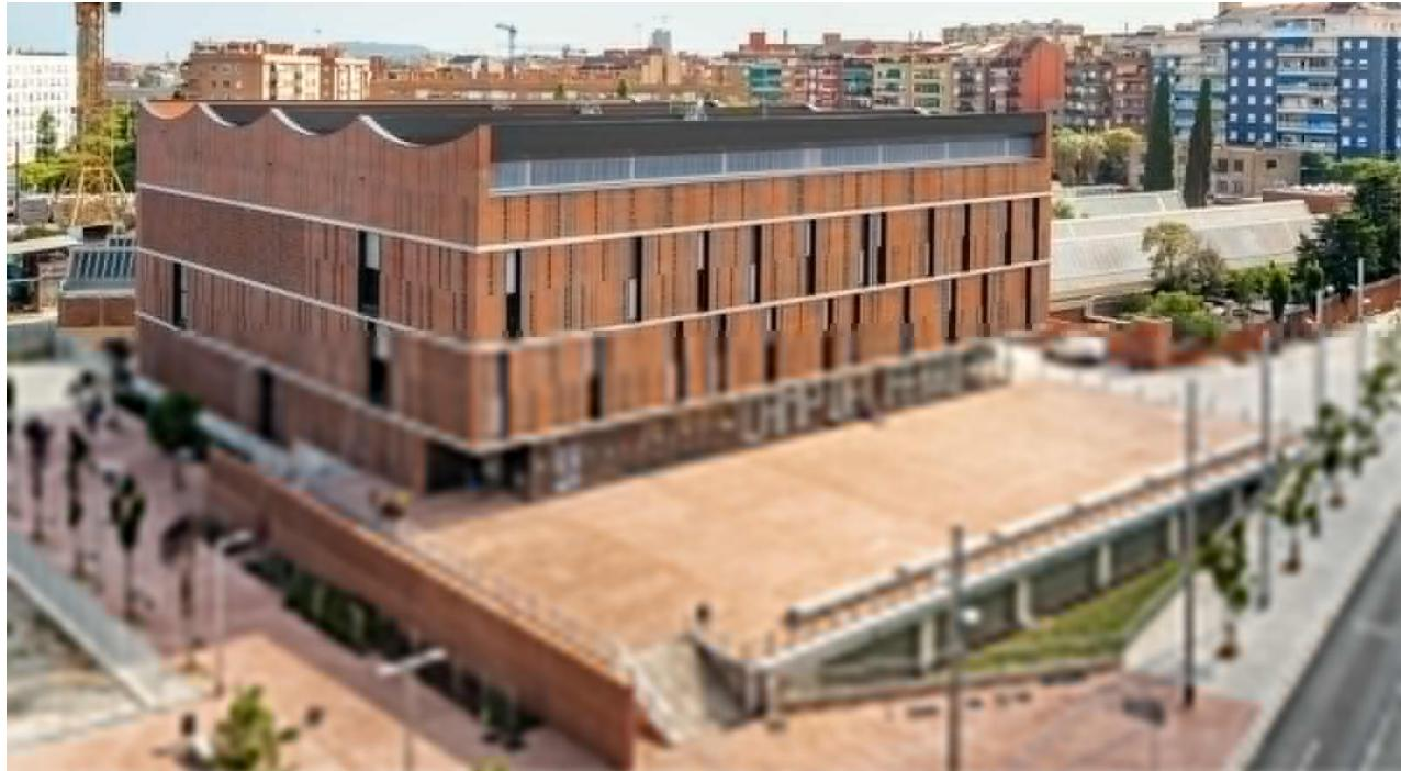
The density of the location, the limited dimensions of the site and the large scale of the brief—the problems tabled by the commission—are counteracted by a useful design solution that consists of semi-undergrounding the facility. Decisions such as the volume of the building, the use of lattice walls for solar protection and the existence of cross ventilation serve to minimize energy requirements and earn LEED Gold certification.
